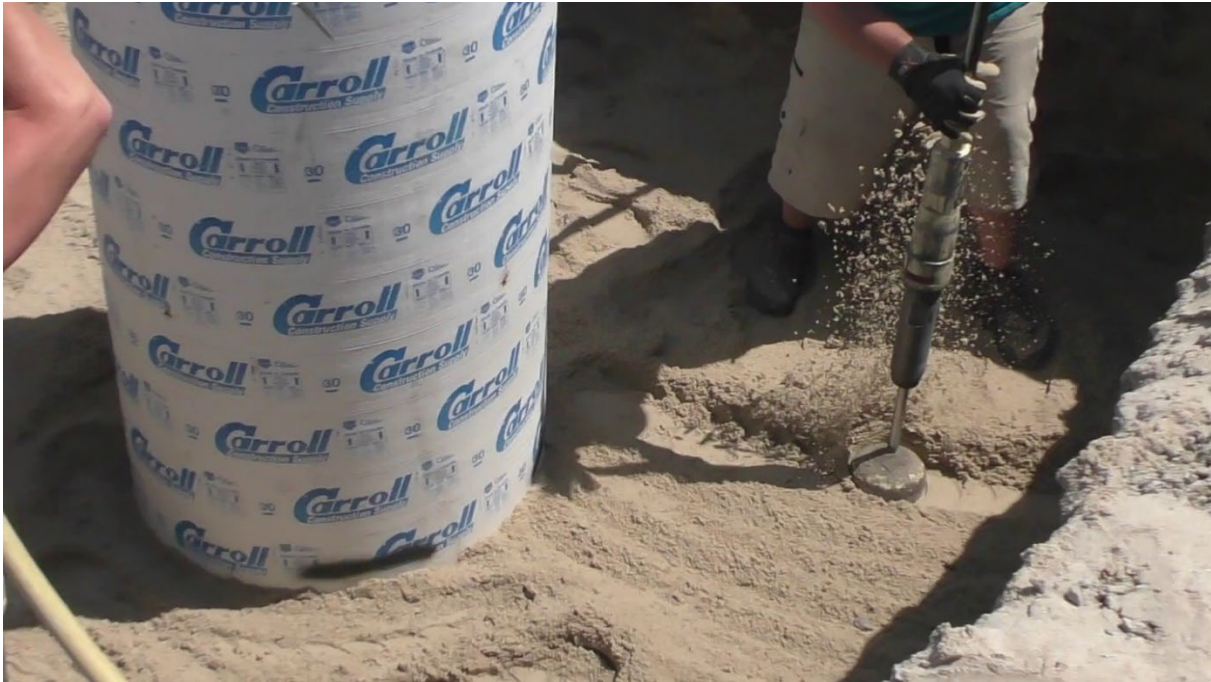
Figure 5.7 Sand Compaction In-Progress, Test No. AKLP-1
