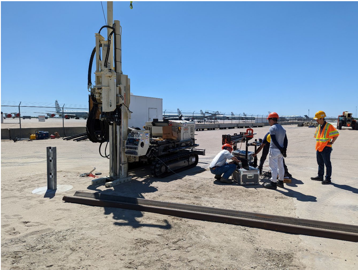
Figure 5.8 GeoProbe Preparing for Soil Testing, Test No. AKLP-1
