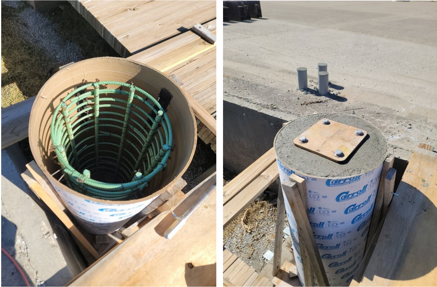
Figure 7.20 Construction Photographs, Test No. AKLP-5
