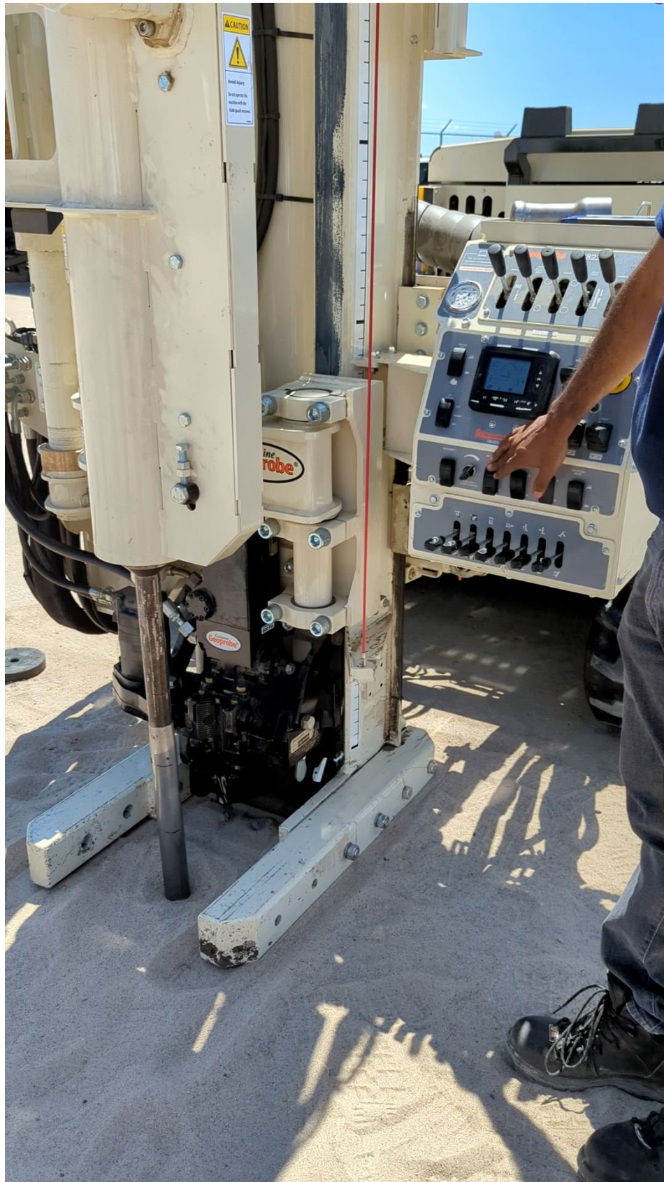
Figure 5.9 GeoProbe Sampler for SPT Testing, Test No. AKLP-1
